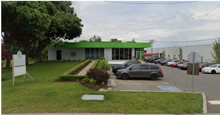
8125 Dixie Road, Brampton
